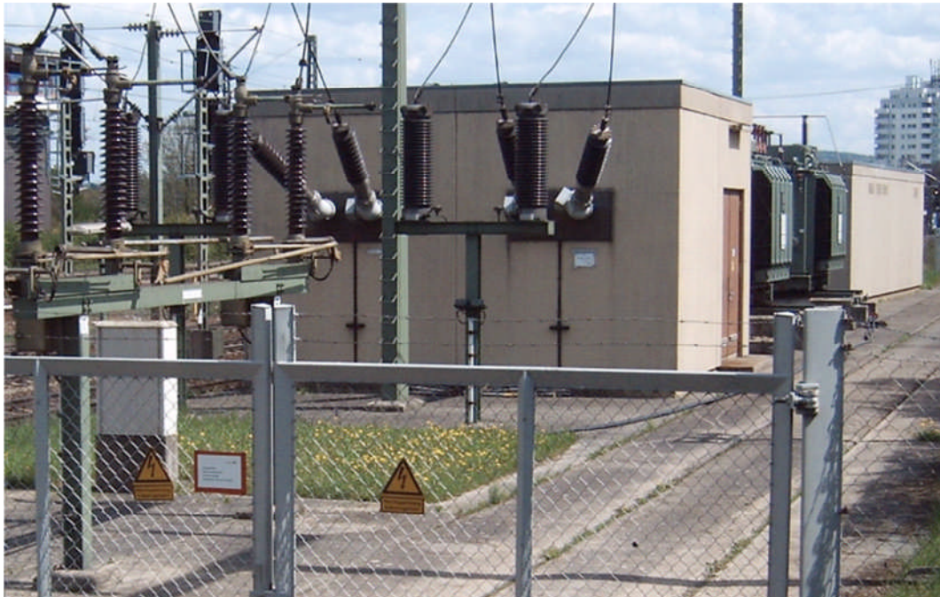
Figure 11: Circuit Breakers
